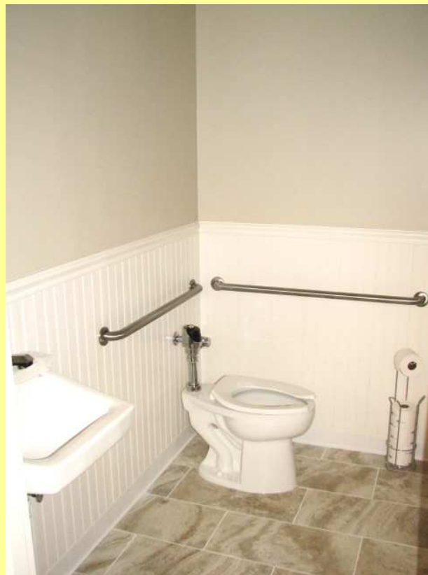
The old mop closet is a new handicapped-accessible bathroom.
