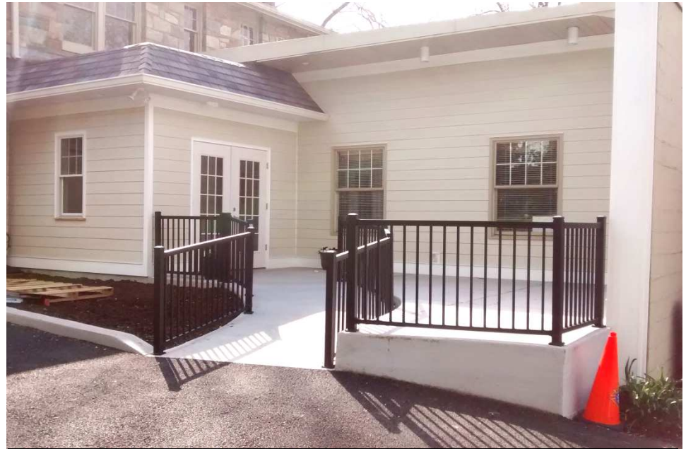
The new side entrance to Cantrell Hall at the Mansion
